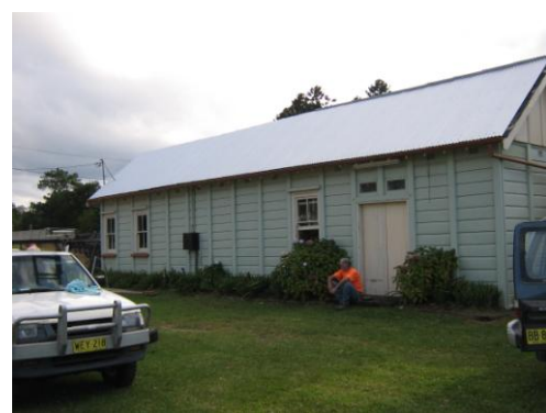
Lowanna Station showing the completed new roof.
