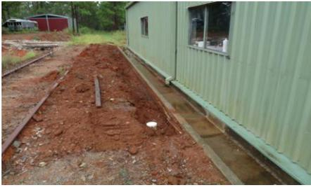
The excavator has been busy since it has come down from Lowanna clearing soil and debris, digging drains, clearing stumps in the cottage grounds and making a culvert. The excavator will head back up top to begin construction of our shed at Lowanna.
