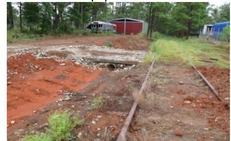
Thanks to the efforts of Colin Sambrook and David Page the mysterious water entry into the crib room when it rains (but it floods only sometimes). What it turned out to be was ground water being forced up through cracks in the concrete. A trench has been dug with the excavator outside the cement drain. We still have to get hold of some agg line and gravel and some helping hands to finish the job!
