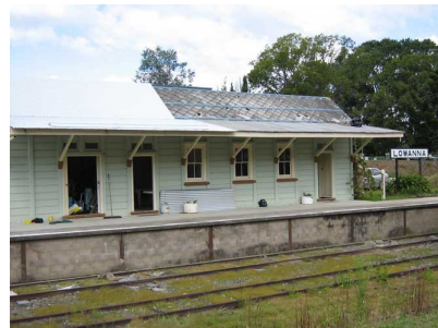
Showing the old and the new roof
